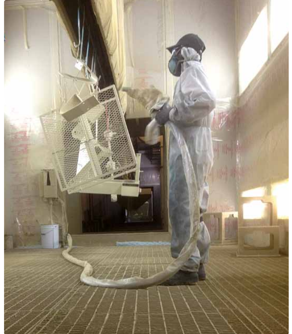
Second anti-corrosion coat and top coat
